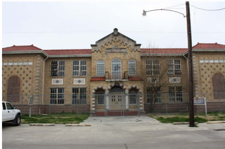
Maumus Art Center. taken by FEMA's SHPO Liaison. 2011
